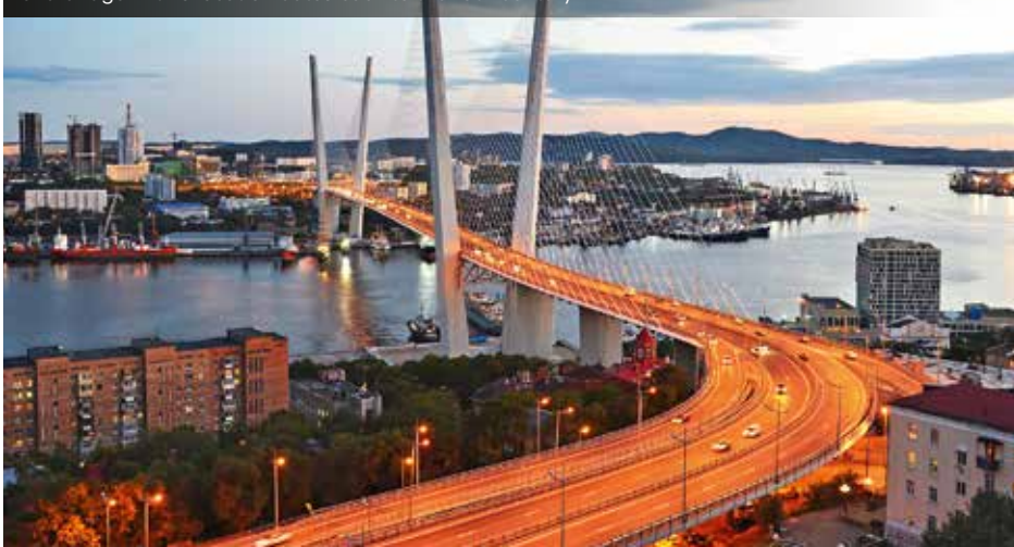
A cable-stayed bridge spanning the Golden Horn Bay was constructed in the city in 2012, even though the concept of a bridge in this location dates back to the 19th century
